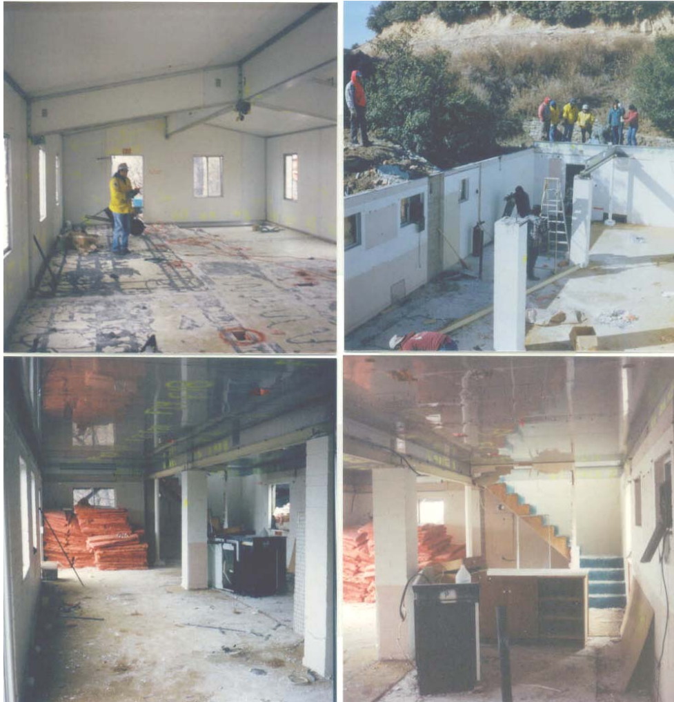
WICKIUP-UPSTAIRS AND DOWNSTAIRS BEING DEMOLISHED
