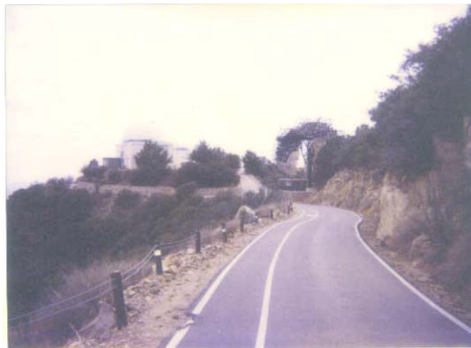
PAVED RIDGE ROAD
