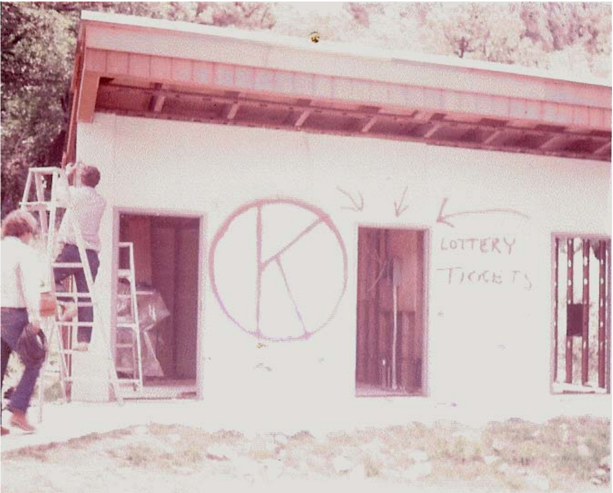
THE BOWL RESTROOM UNDER CONSTRUCTION
