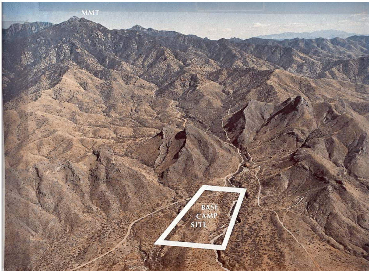
AERIAL VIEW OF THE PROPOSED BASE CAMP SITE LOOKING EAST
